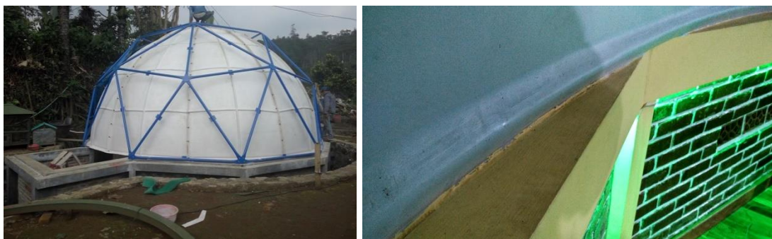
Fig 7. Fiberglass inner dome and sealed connection between the inner dome and the wall (Source: Owner documentation, 2018)
