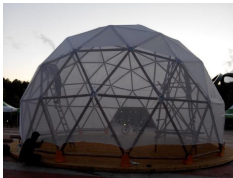
Figure 2. Built geodesic dome in World Bamboo Festival 2015 (Source: Project documentation, 2015)
