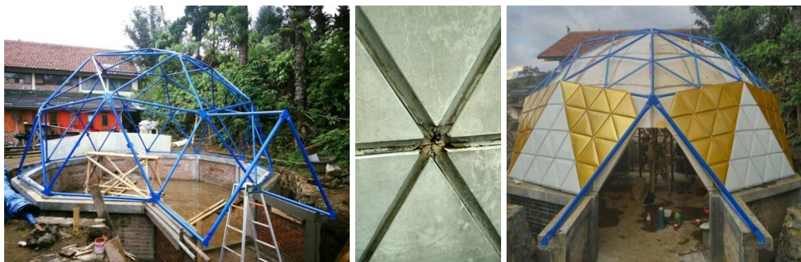
Figure 6. Steel frame for the entrance, detail of enamel roof, and additional struts (Source: Owner documentation, 2018)
