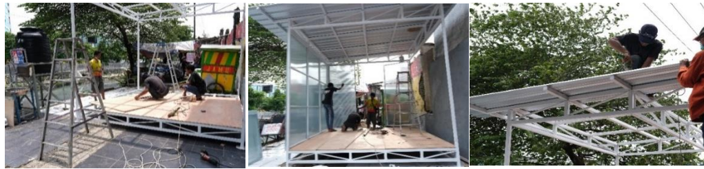
Figure 6. Floor, roof and wall covering installation
