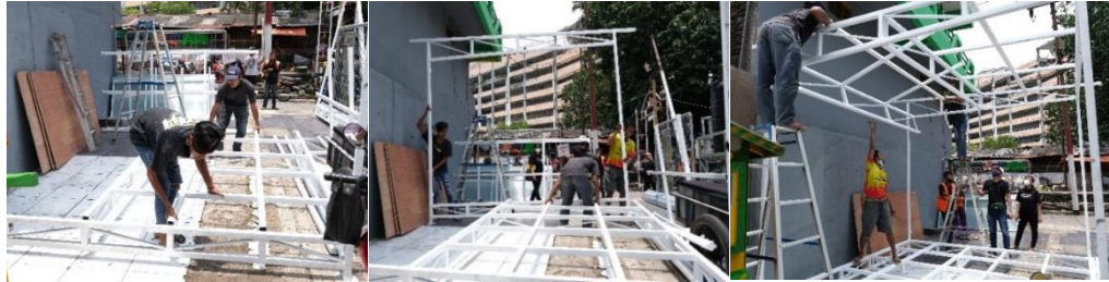
Figure 5. Floor, column and roof structure frames installation
